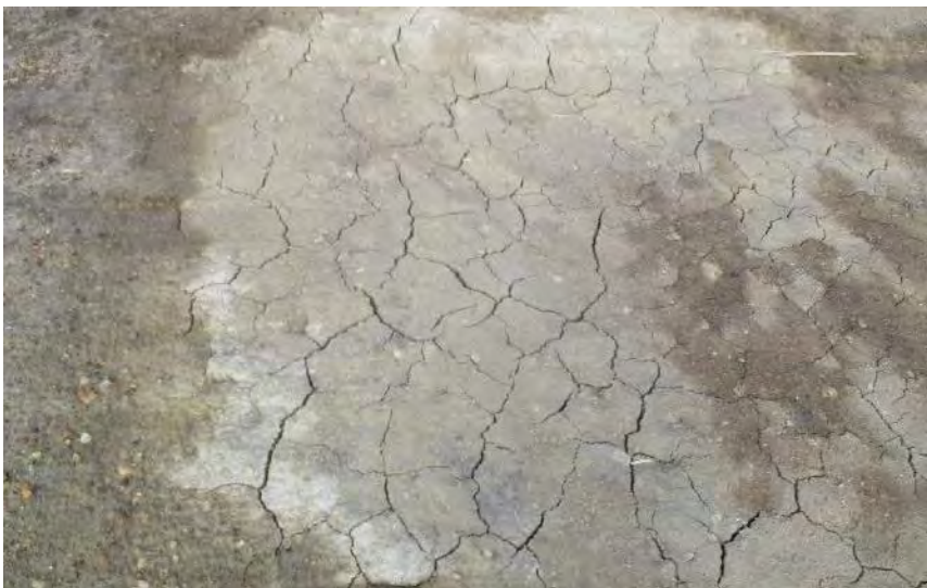
Photograph showing a closer view of soil cracks with slight salt crusts on site.
