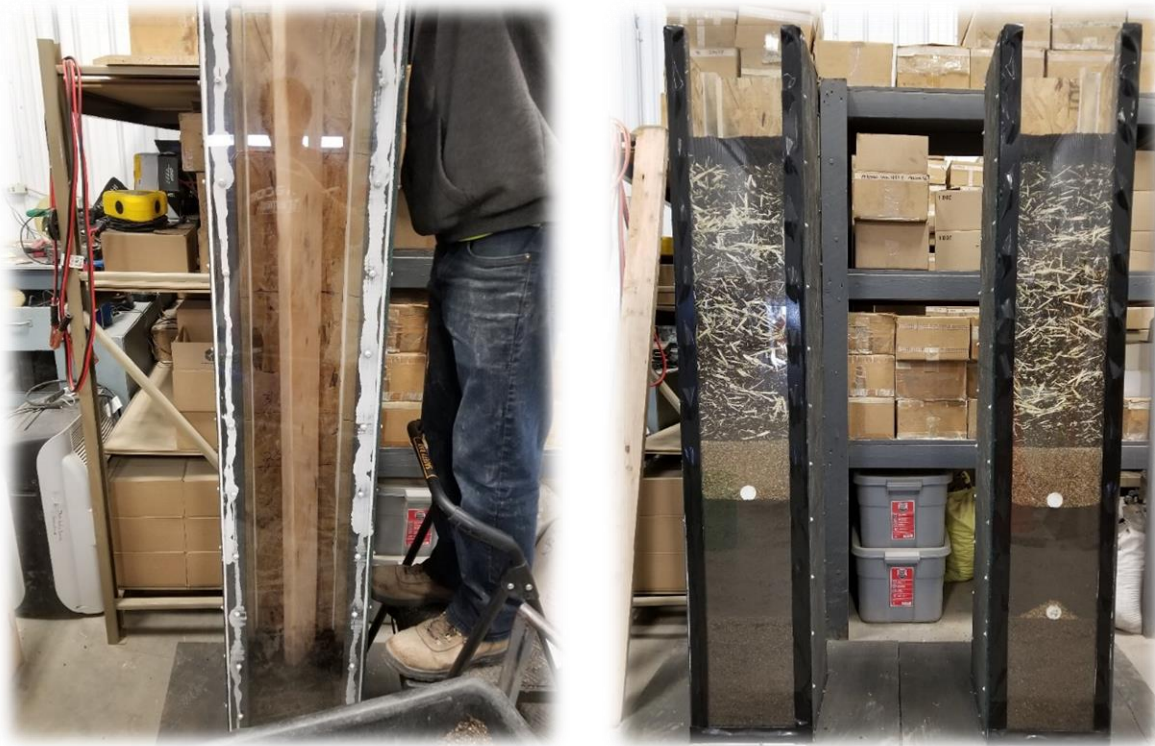
Images 12 & 13: Attaching the Plexiglas in the front of the columns and the finished columns.
